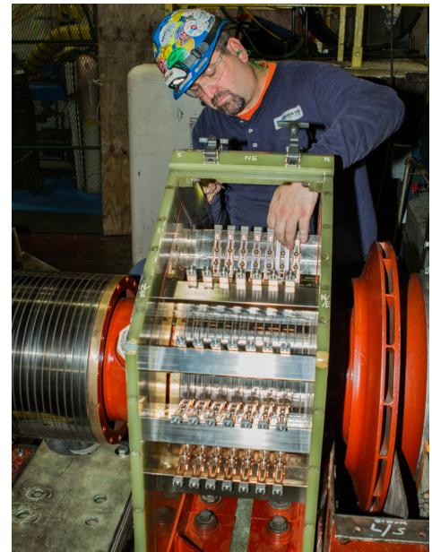
Cutsforth™ Technicians come on-site to install and calibrate your new rigging and inspect other excitation conditions
