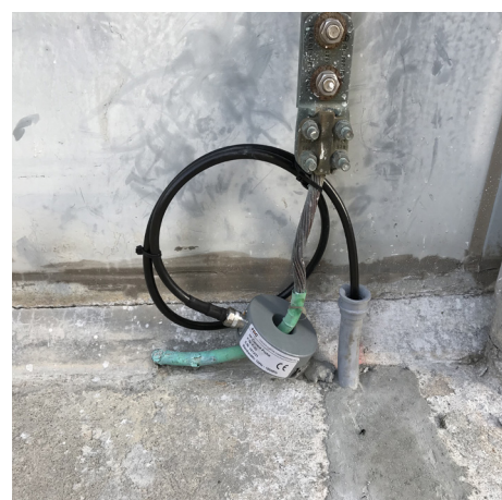
Radio Frequency Current Transformer (RFCT) installed on the Frame Ground; usually coupled around the Generator to Neutral Ground connection.
